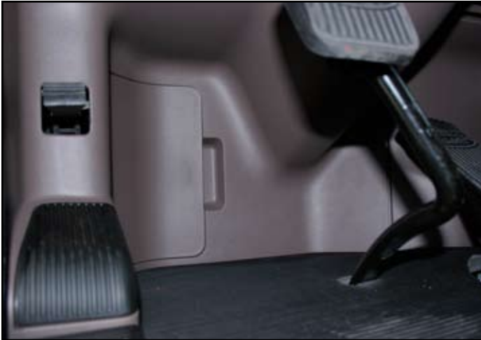
Kick Panel Door Concealing Fuse/Circuit Breaker Panel
